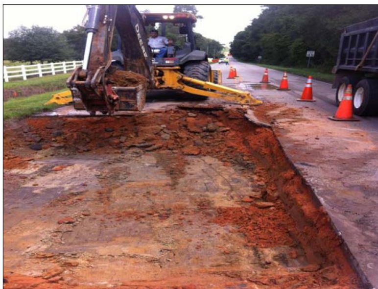
Asphalt Road Maintenance
