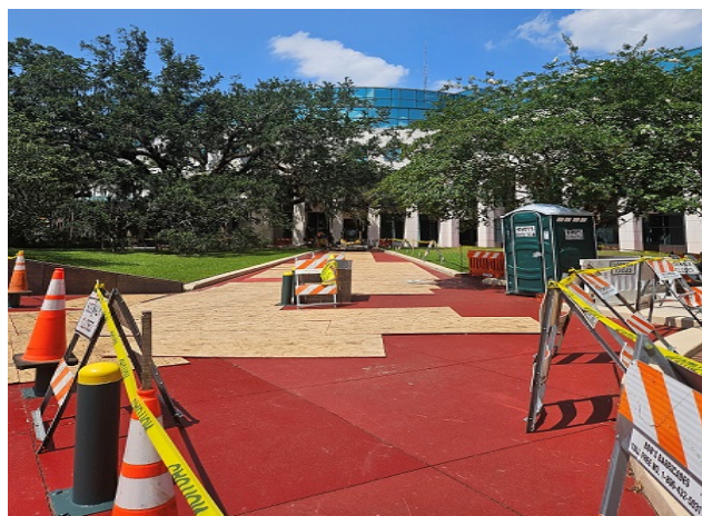
Building Infrastructure and Improvements - Courthouse Plumbing Repair
